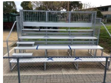
Illustration 11 Grandstand adjacent to Technical Bench area - 1.5 metre distance markings
